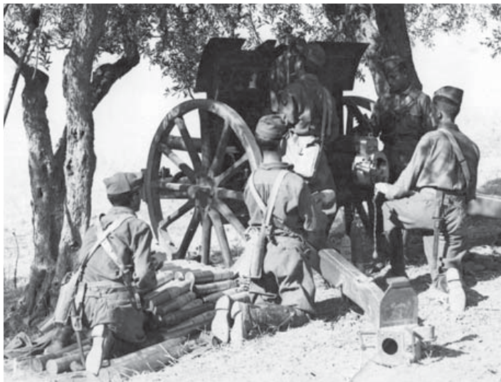
CTV gunners crew a 75mm cannone da 75/27 Modello 11 . This pre-World War I field gun would remain in Italian Army service well into World War II, and was even pressed into service by the Germans in 1943–45 as the 7.5cm Feldkanone 244(i) . (AdeQHA)
