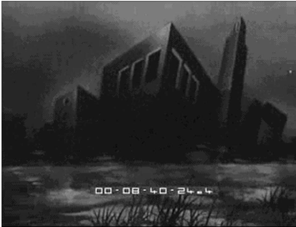
Figure 4 Sabaudia rising over the marshes. Source: B0547.
